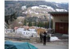
District heating plant in the Alps, Italy 550 kw
